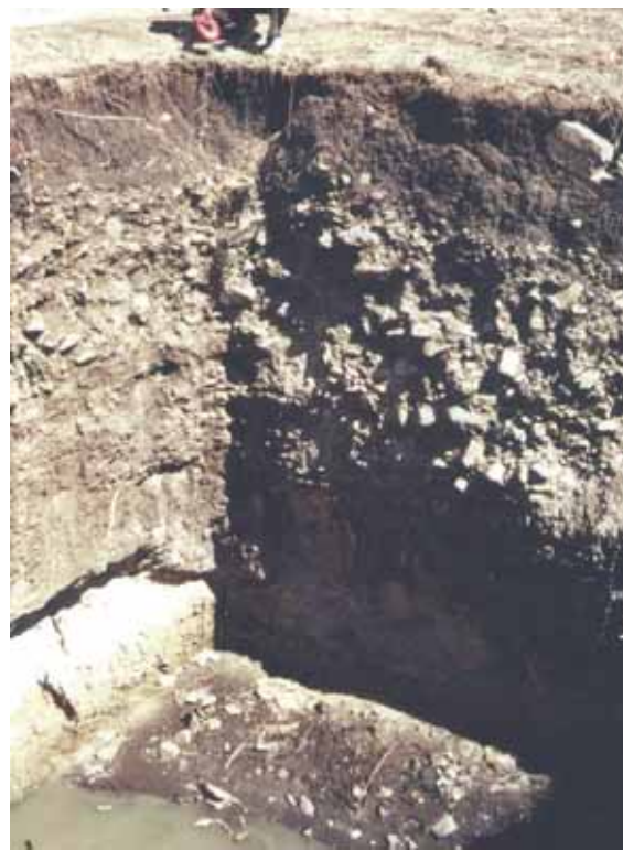
Private dug-out well
