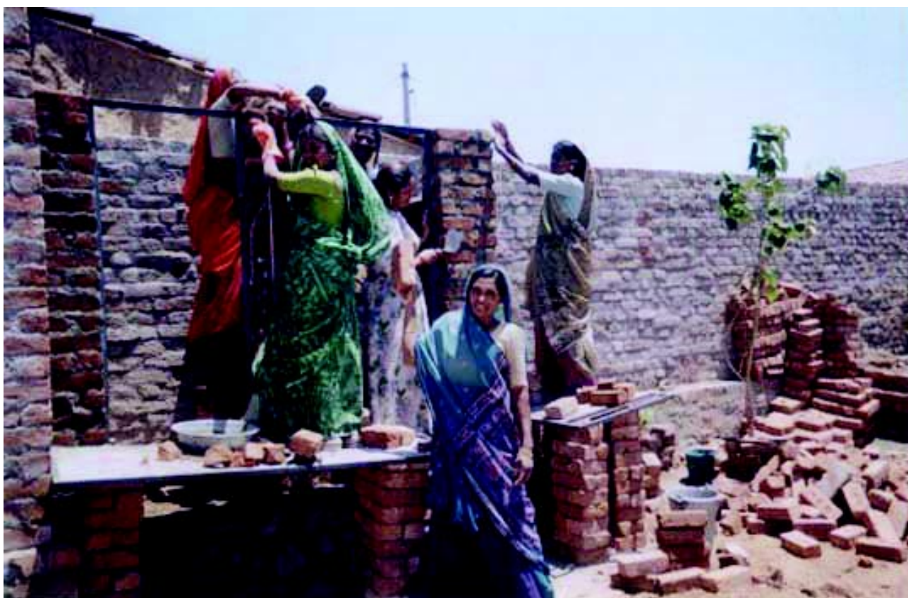
Women at masonry work
