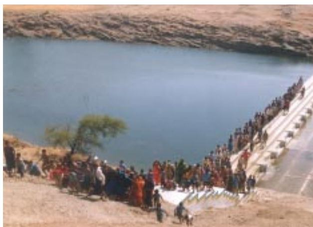
Check dam at Borkhedi
