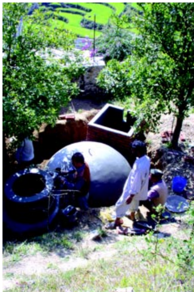
A biogas unit under construction
