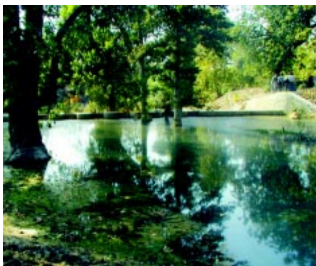
Sitapuri check dam
